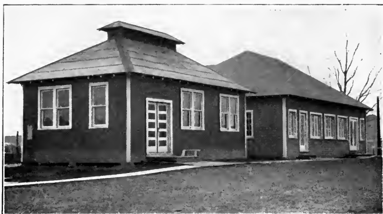
The Nela Camp Dining Room. It was equipped as a temporary hospital for the Defense Section during the Influenza Epidemic
